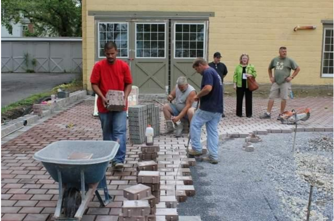
Volunteers put water permeable eco pavers into the courtyard at Perkins Center for the Arts in Collingswood. / JAN APPLE/For the Courier-Post
